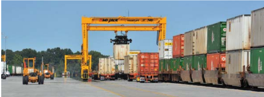
Six railyards—including Norfolk Southern's new Memphis Regional Intermodal Facility—offer the combined capacity to lift more than two million intermodal containers per year.
